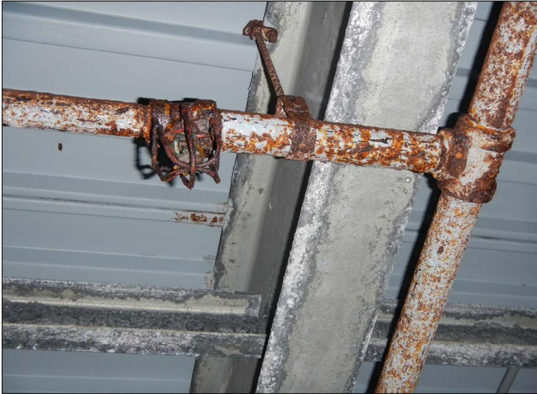
Corroded Sprinkler Pipe
