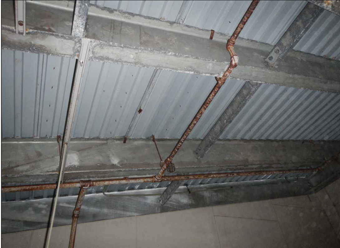
Corroded Sprinkler Pip
