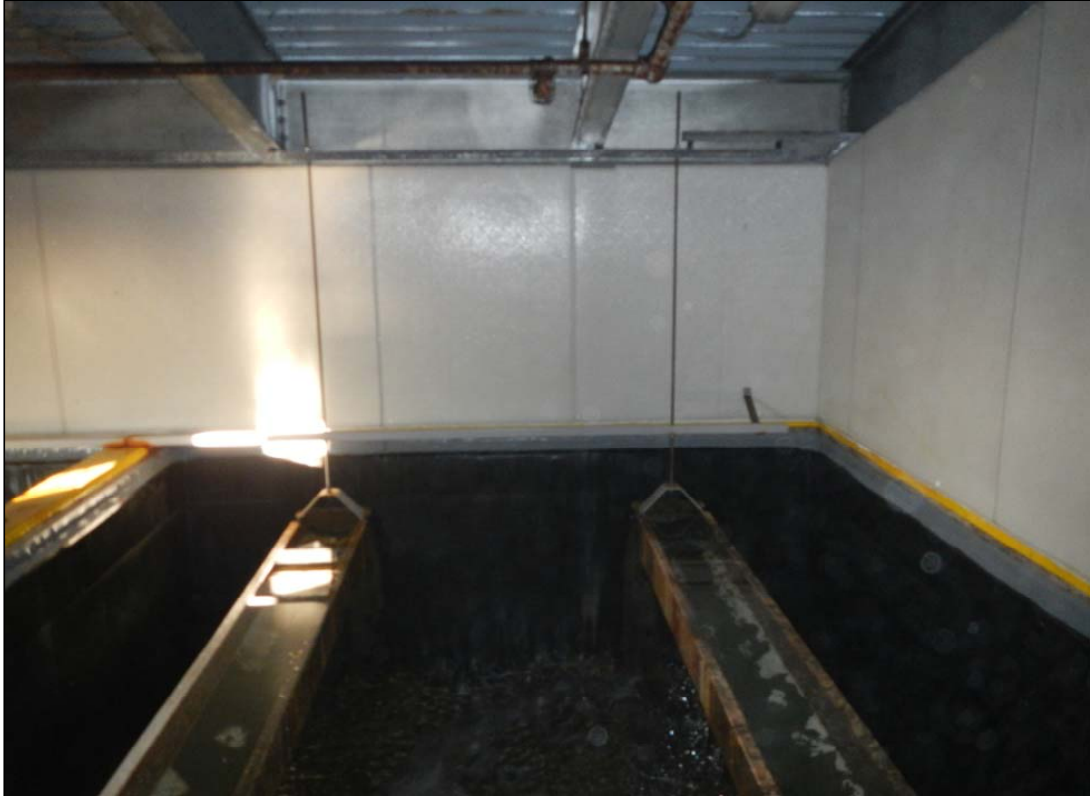
Sprinkler Pipe Over Seawater Filter Tank
